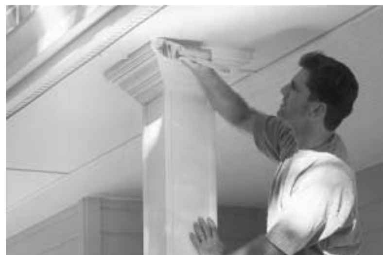
Paint the fascia boards, gutters and eaves first.
